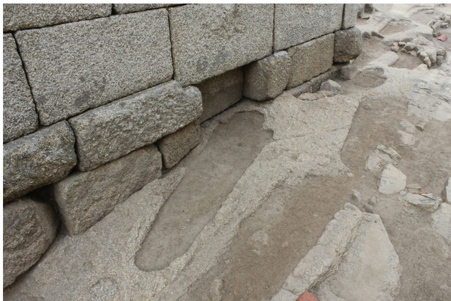
Figure 8. Re-entrance of the Church's foundations so as not to hide a rock-cut tomb.
