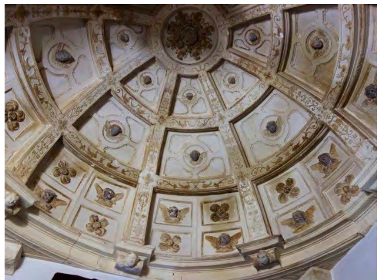
Fig. 18 - Chapel of the church of Cumeeira, Penela, late 16 th century. @ Maria de Lurdes Craveiro
