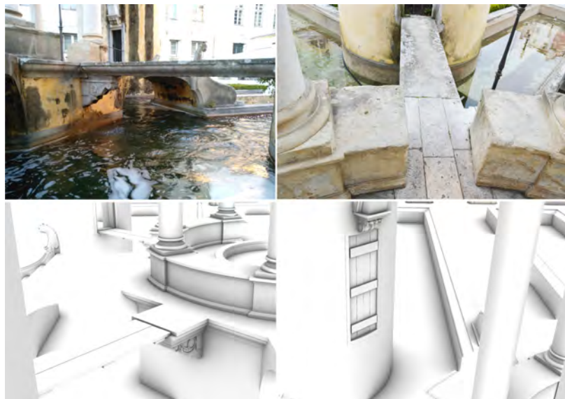
Fig. 18 [a; b; c; d] - Details of the Manga tempietto and conjectural reconstitution of the drawbridges, by Miguel Alberto Pedrosa.
