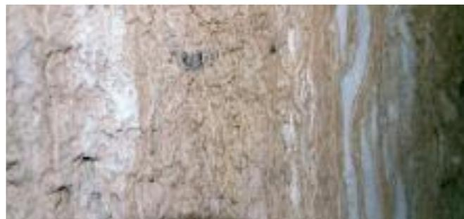
Fig. 5. Worm cast type structures visible at Ambel beneath a previously damaged roof section
