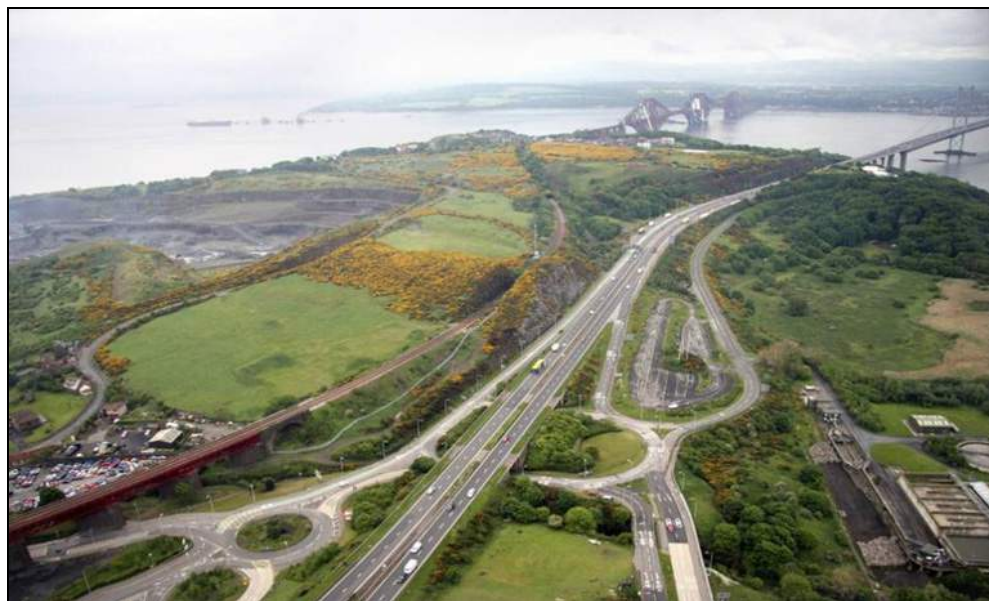
Fig. 14 – Acesso Norte a Forth Road Bridge (Menard).
