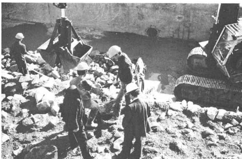
*Fig. 4 — Aterro experimental com enrocamento argamassado*
