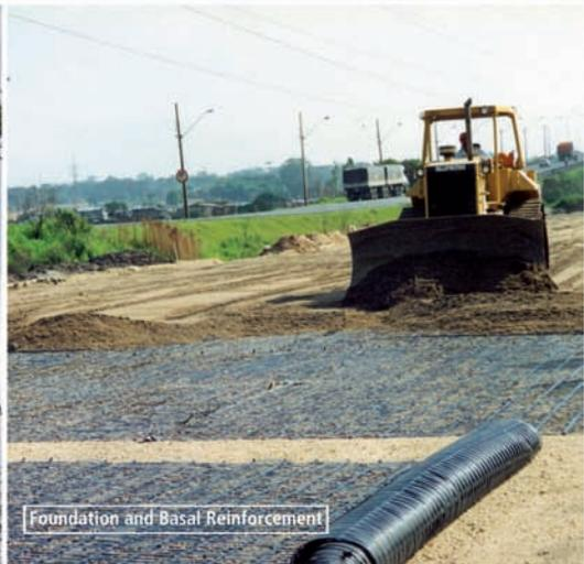
Foundation and Basal Reinforcement
