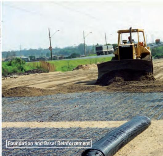
Foundation and Basal Reinforcement
