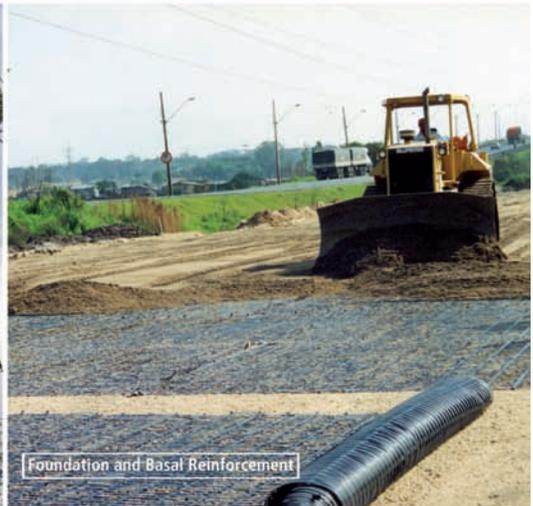
Foundation and Basal Reinforcement
