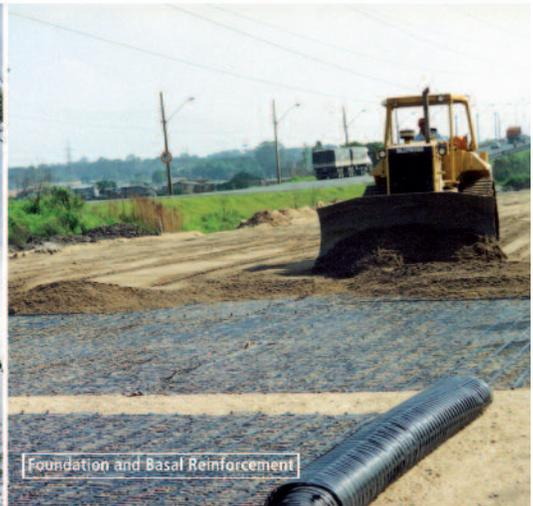
Foundation and Basal Reinforcement
