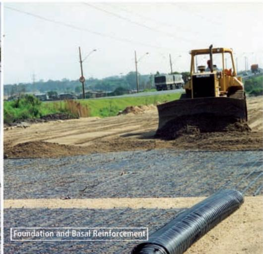
Foundation and Basal Reinforcement
