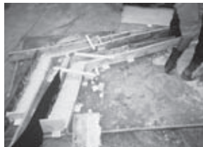
2. Concrete casting/testing, Architectural Association.
