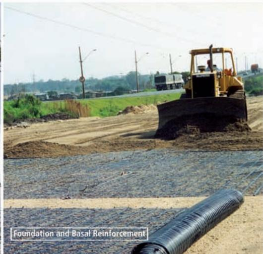
Foundation and Basal Reinforcement
