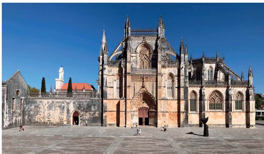
Fig. 1. Batalha monastery’s west façade. Photograph: Pedro Redol.
