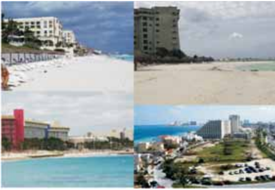
Fig. 26: other views of the built environment that is typical of the hotel resort area in Cancun. The views on the left of this figure show several hotels built on the water side of the dune of the original island and the use of retention walls to allow for landscaping and even sand to be maintained on the waterfront of these buildings. The pictures on the right show buildings on the northern man-made land bridge linking the original Cancun Island to the mainland, which has no dune allowing for buildings to be built even closer to the waterline and at lower elevations (as low as only 1.5 to 2 m above mean sea level) with respect to mean sea level.
